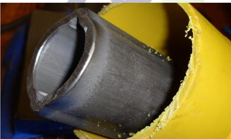
Figure 45 burrs removed with a file, grinder and power wire wheel.
